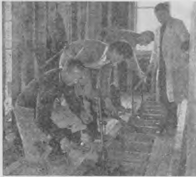
Cramping a floor.
