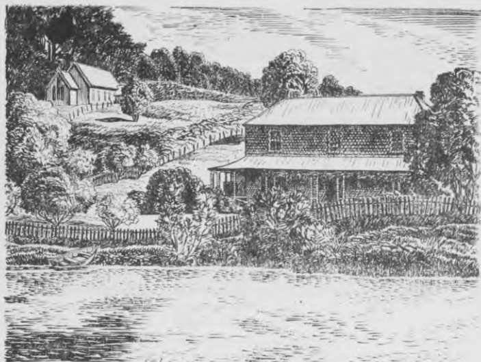
James Kemp's house and the Anglican church.
