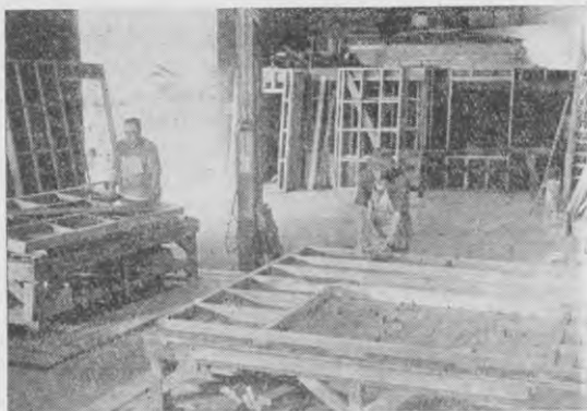
Two of the jig tables with the panels being assembled.
