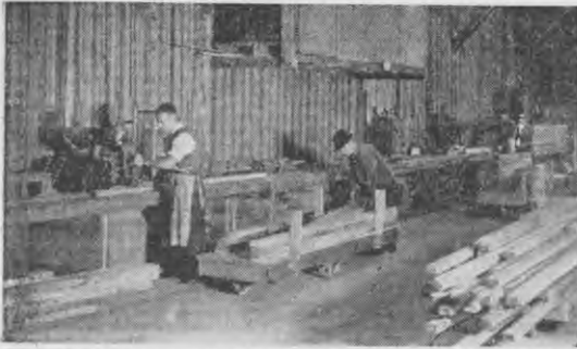
The first saw ; and the timber proceeding to the second saw. The numbered patterns can be seen hanging on the wall at the rear.
