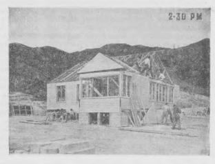
II. The trusses are all up and the first end piece has gone up. The two men on the left of the sun-porch are putting on the lower weather-boards where the bottom of the panel joins the flooring.
