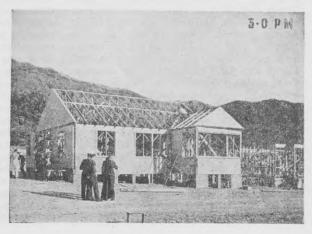
12. The exterior shell complete, including entrance porches at side and rear, with the first priming coat applied at the factory. Erection time, including the foundations, was fifteen hours.
