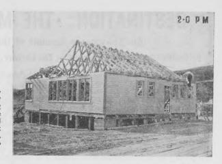
10. Another roof-truss coming up. A start has already been made on the hip covering the front sun-porch. Note that the main prefabricated trusses continue straight through regardless of the hip. This gives extra strength to the main gable.
