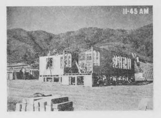
7. The outer shell is complete except for the sun-porch panel. You can see the joins where the panels meet. These will be covered with battens.
