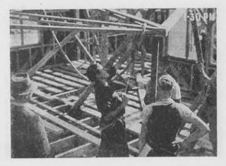
9. Here we see how the rooftrusses are pushed up one by one until the seventeen comprising the main gable are in position.
