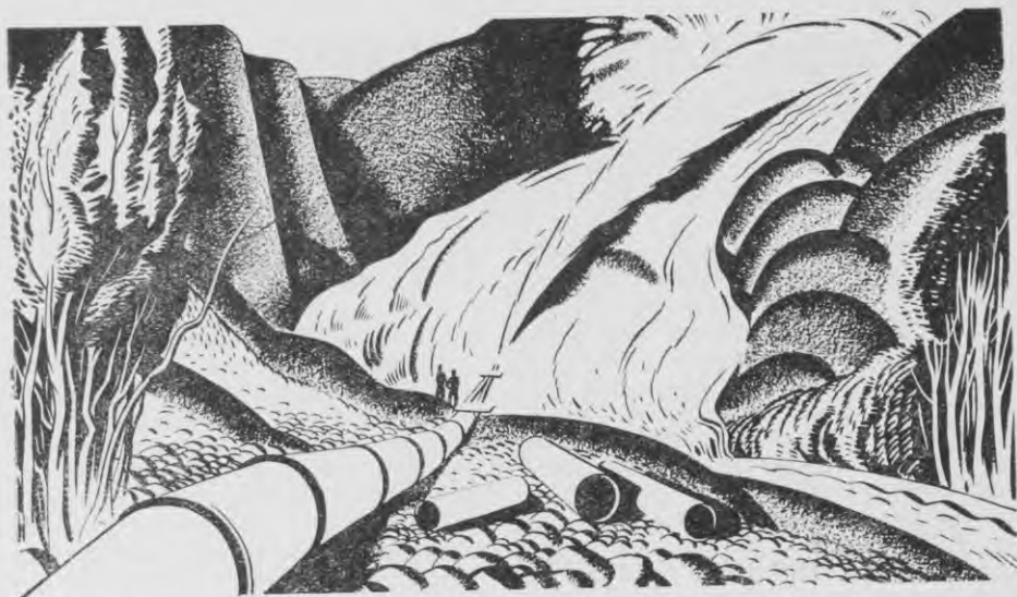
A modern sluicing claim. The large pipe-line in the foreground is carrying water up to the cliff face. In the bottom right-hand corner can be seen the race down which the water and the gold-bearing wash travel.
