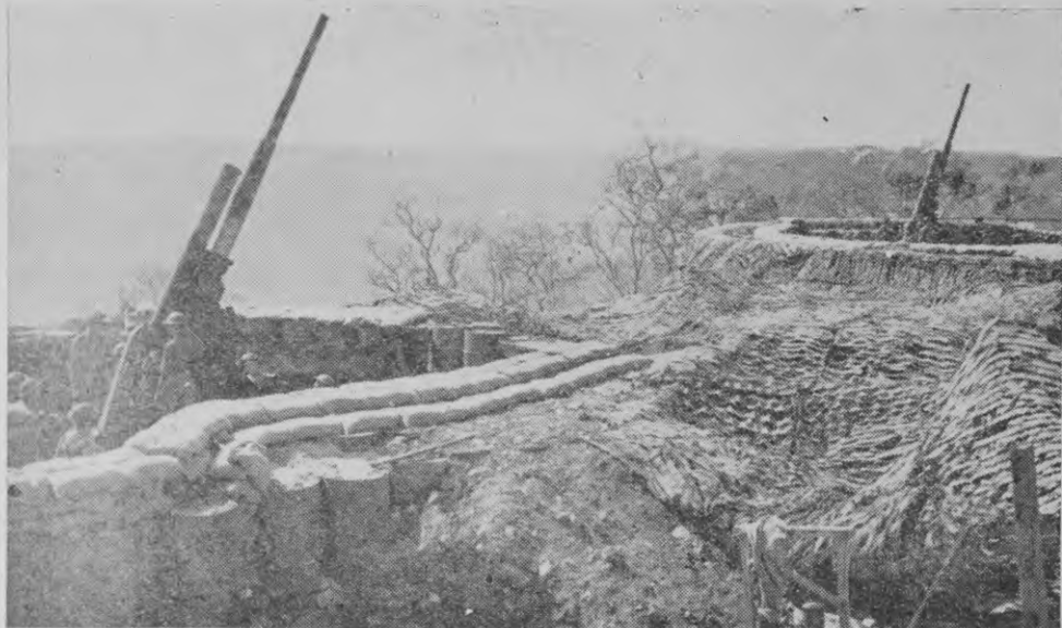
ACK ACK IN AUSTRALIA.—Guns of an Ack-Ack battery near Melbourne. Auckland gunners may be interested to compare the construction of their pits with the ones shown in the picture. Camouflage can be seen on the right.
