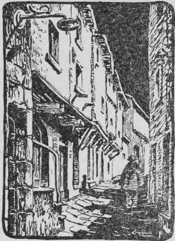
Street Scene in Cortona. Note typical overhanging upper storey
