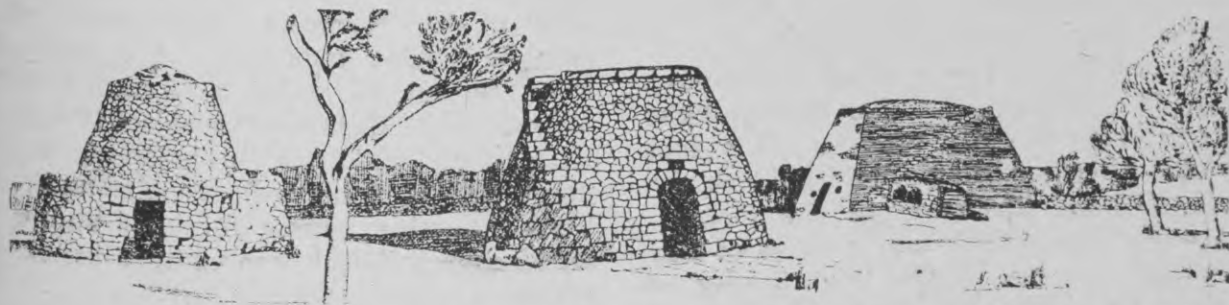
A composite picture of three Trulli of the Salentino district. Interesting types are the galleried Trullo (left) and the square or truncated pyramid Trullo (right).
