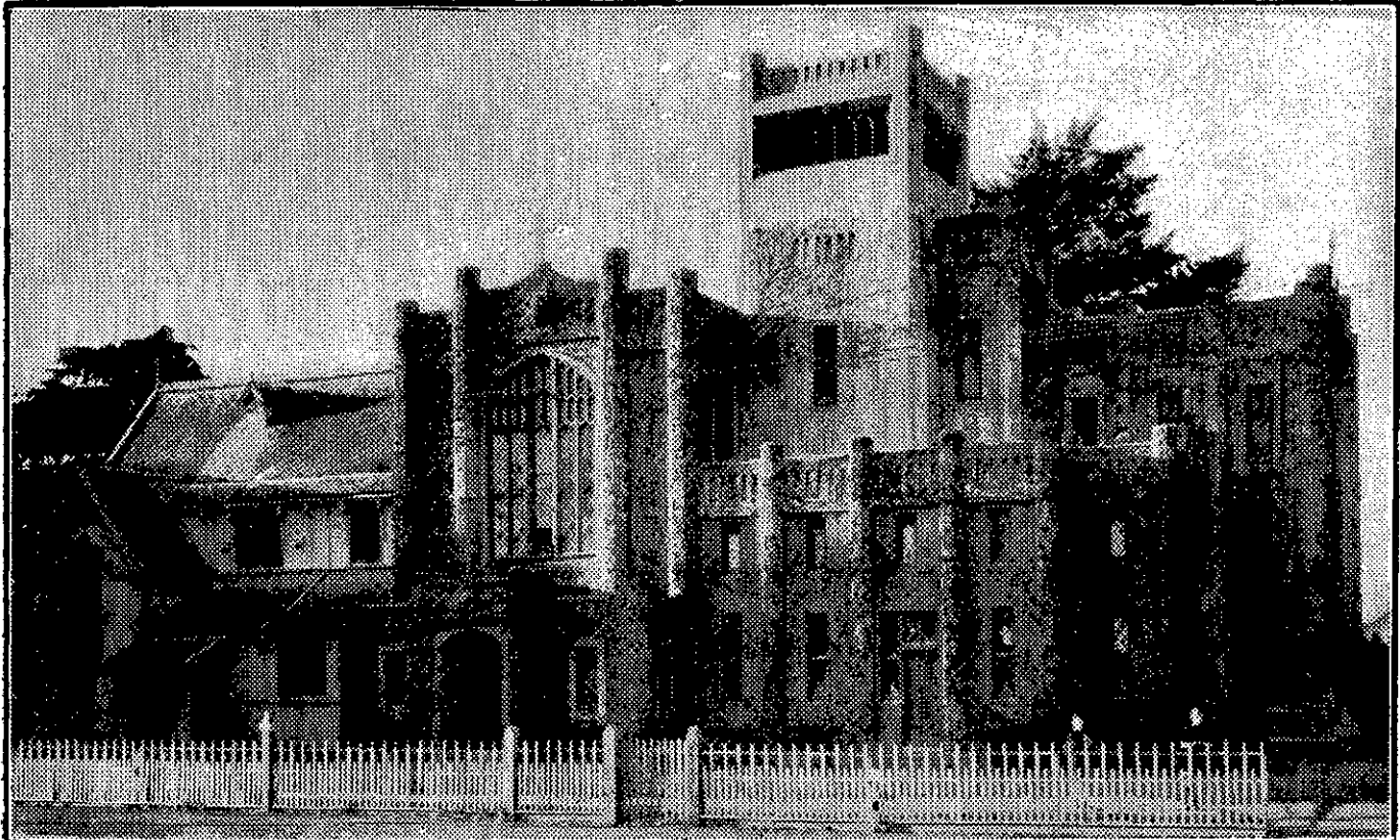
ST. MATTHEW'S CHURCH, HASTINGS, AS RE-CONSTRUCTED AFTER THE EARTHQUAKE.
