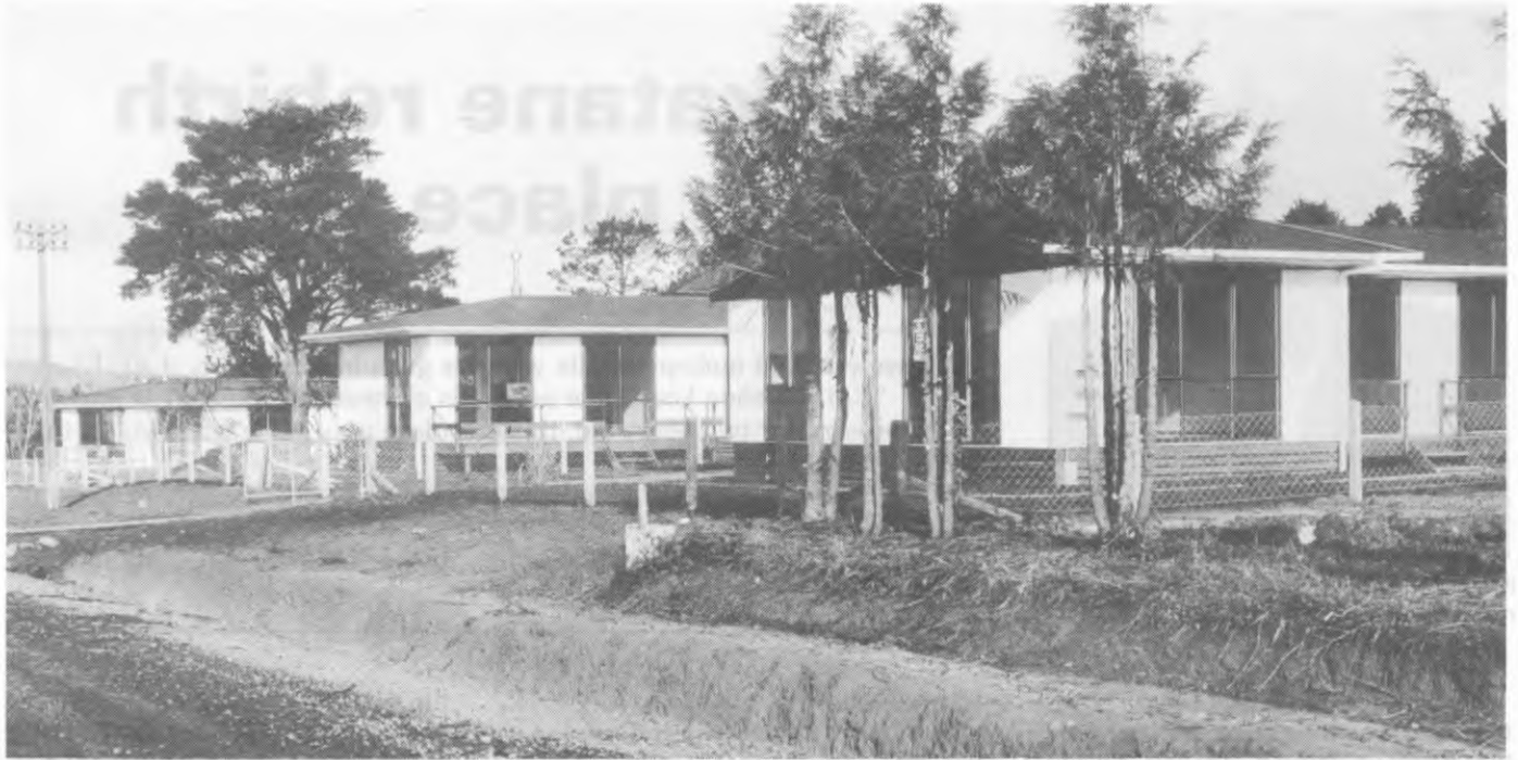
The houses in the Te Horo District — the first to be built in Northland under the Housing Corporation's rural rental housing scheme.
