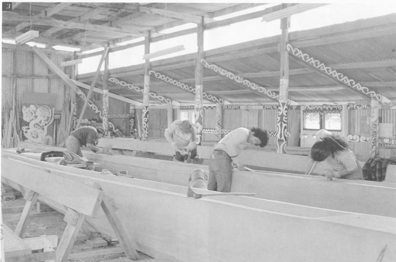
Kim adzes inner hull while older brother Greg adzes the other 1. Kim uses axe to block cut inner hull 2. Unpaid work team, Greg, Robert, Alan, Dave. Kim took the photo 3. Art of the adze. Greg remembers Kohe Webster teaching him adzing on an old power pole in 1976. Rua taught him in 1978 the broad blade adze art 4. Second hull bow shape 5.
