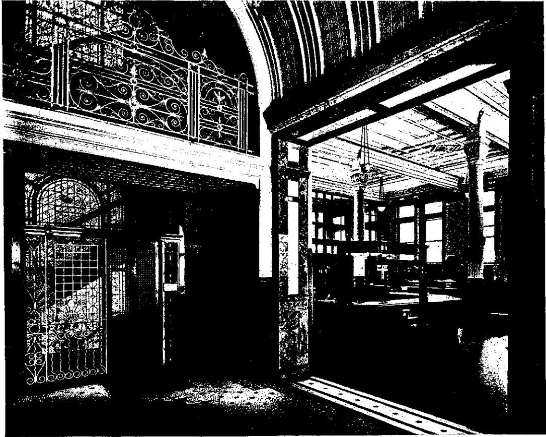
Messrs. Burns, Philp & Co.'s Sydney Offices.—Northern Side. Ground Floor. Entrance View.
