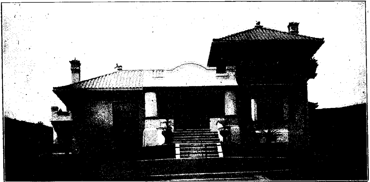
No. 1. A Californian Bungalow, Cement Finished, in Ornamental Mission Style. Plan shown on page 569.
