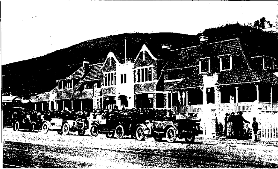
The Ross Home.—New Home for Aged and Needy, by the Presbyterian Social Service Association. Architect: Mr. W. H. Dunning. [Contractors: Messrs. Fletcher Bros.]
