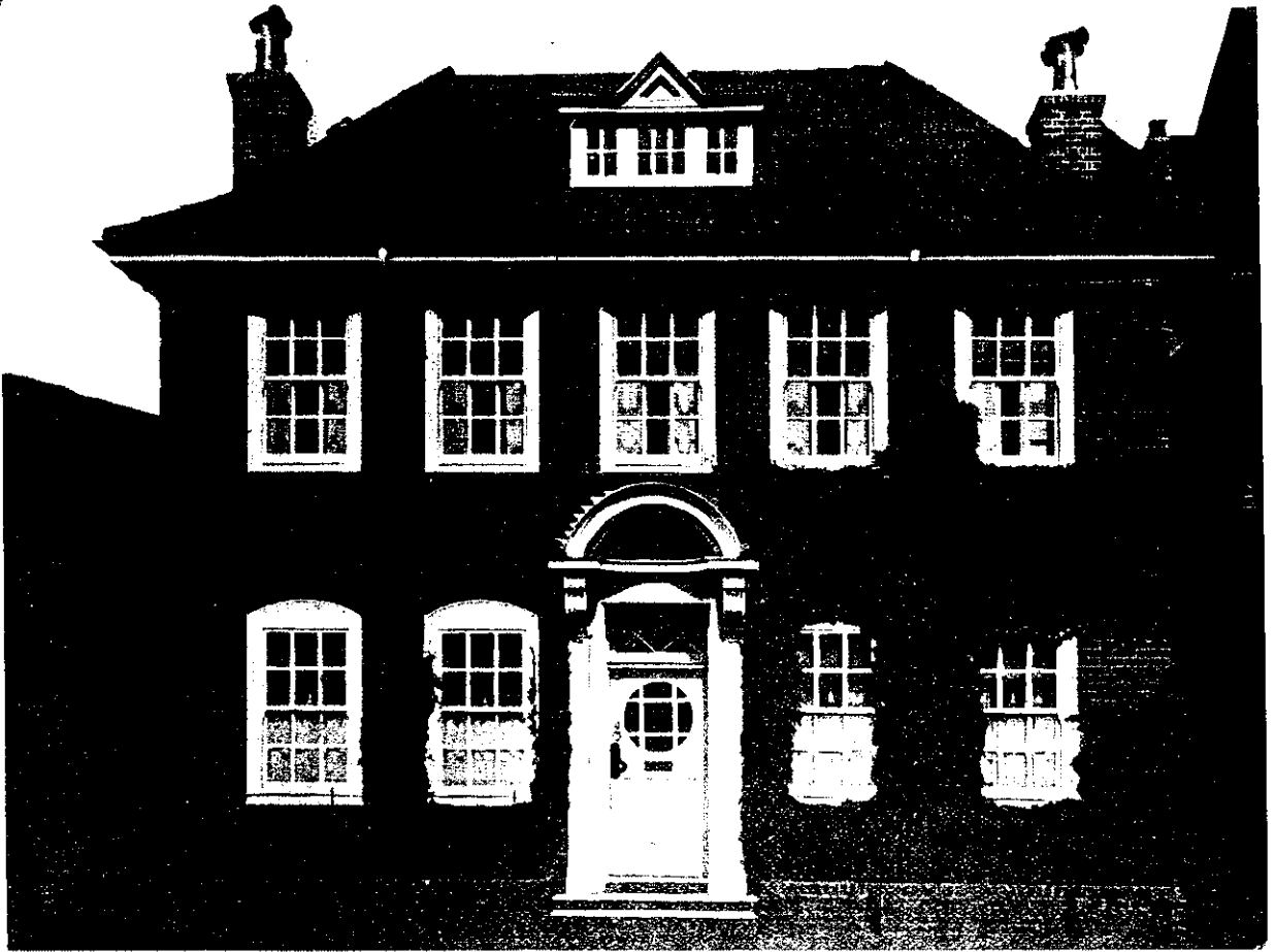
MODERN DOMESTIC ARCHITECTURE.—Doctor's Residence, Wellington W. Gray Young, F.N.Z.I.A., Architect
