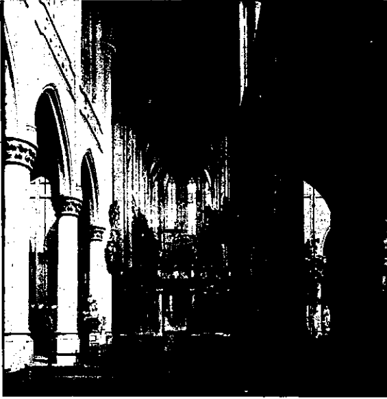
Fig. 7—Church of St. Jacques, Antwerp, shewing Columns with Capitals giving evident Support to the Wall above.
