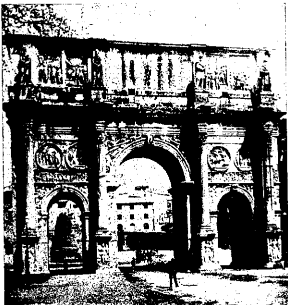
Fig. 5—The Arch of Constantine near the Roman Forum at Rome, shewing Columns used as Decoration.
