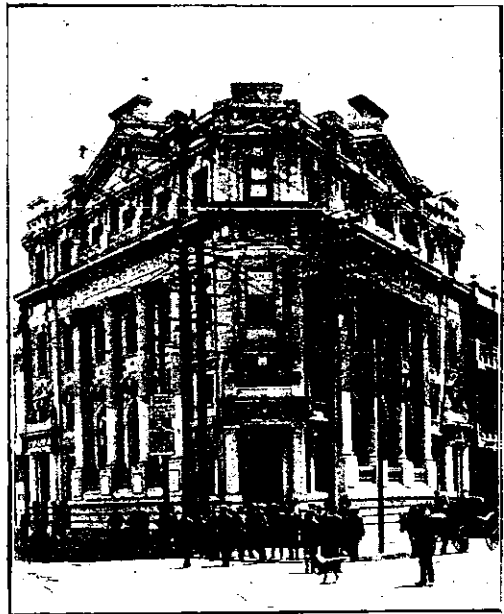
BANK OF N.Z., MANNERS ST., WELLINGTON. Built with Golden Bay Cement.
