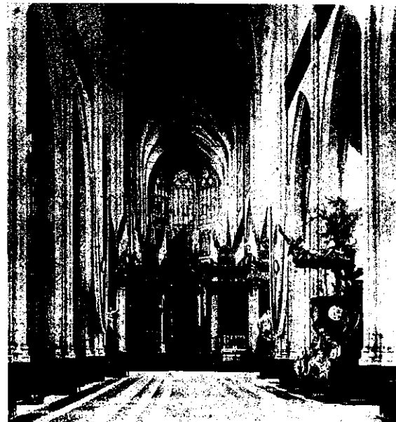
Fig. 8—St. Bavon, Ghent, shewing Diminished Beauty by the Omission of the Capitals of Columns.
