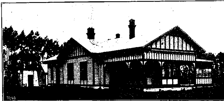
This house, the Residence of Mr. F. Sowden, Aylesbury, Canterbury, was built of Pinus radiata Timber grown on the Property.
