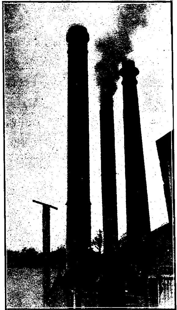
View of Finished Chimney
