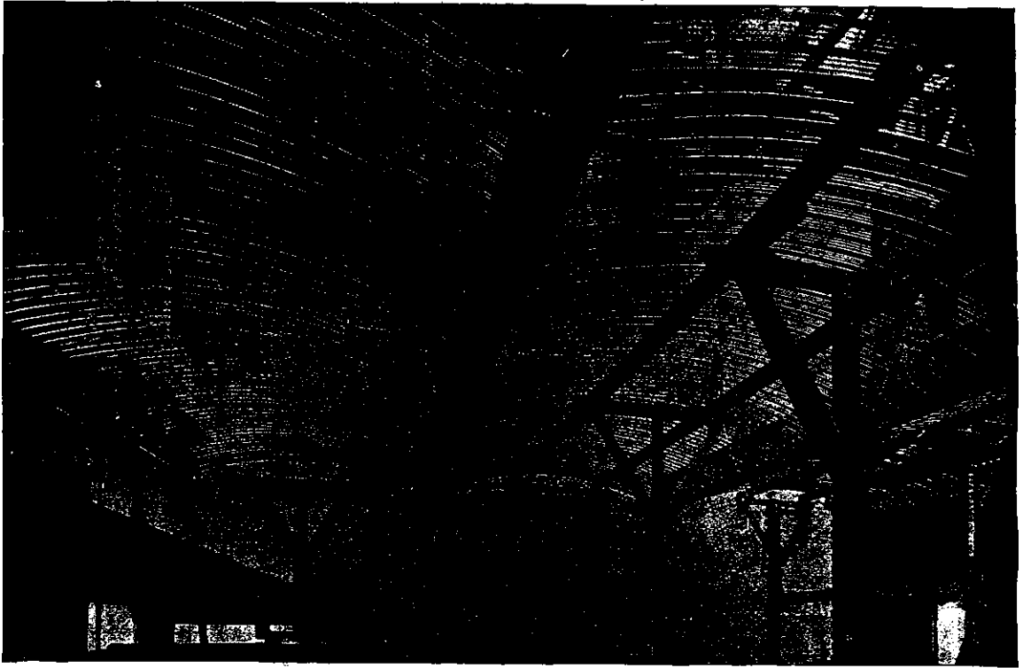
Arched "HY-RIB" Floor before concrete is poured. "HY-RIB" provides in itself the centering and reinforcement.
