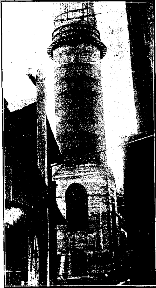
View showing Circular Formes employed
