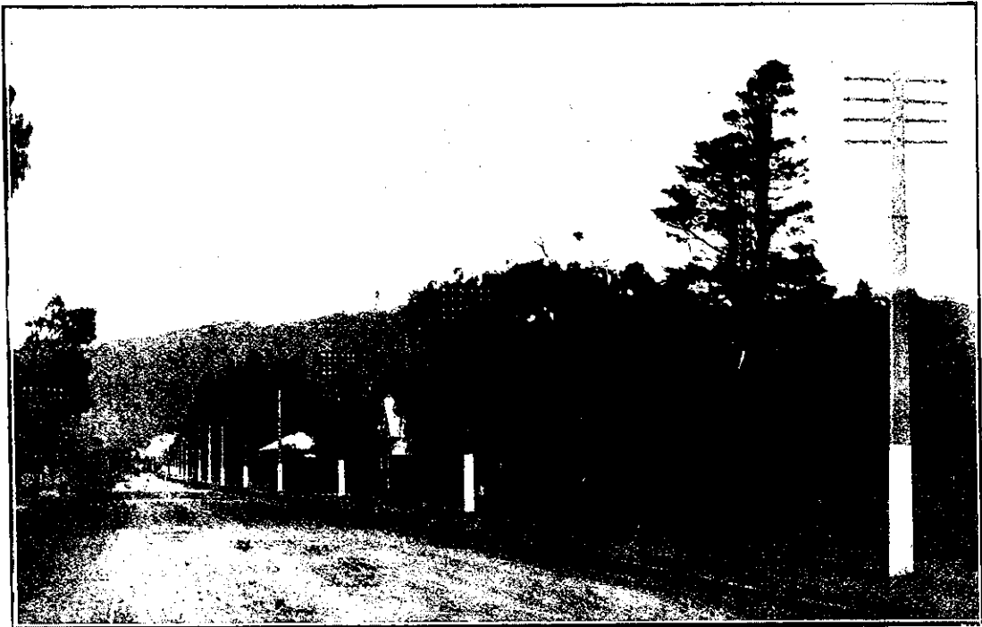
CONCRETE POLES ON THE LOWER HUTT-MASTERTON TELEGRAPH LINE
