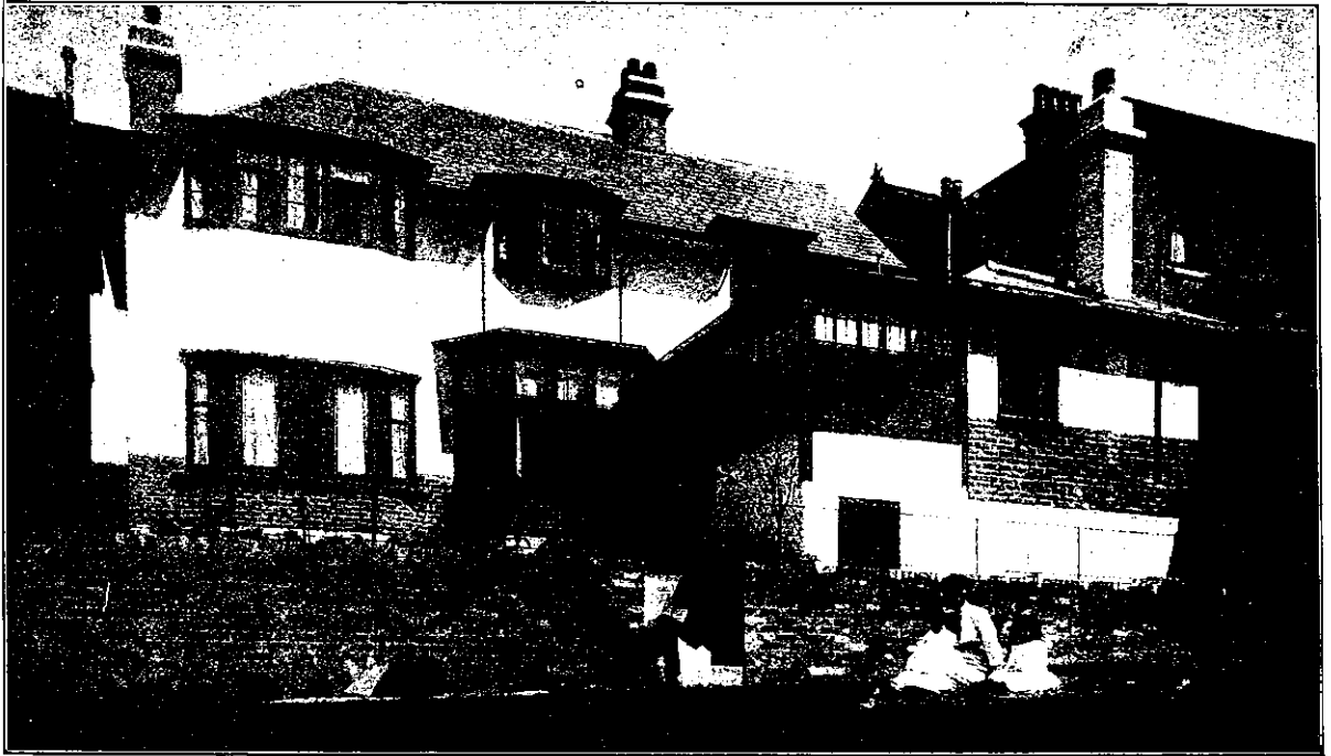
BACK OF HOUSE IN HIGH STREET, DUNEDIN, Showing the advantage of a sunny back aspect. The garden is private, sheltered and sunny.
