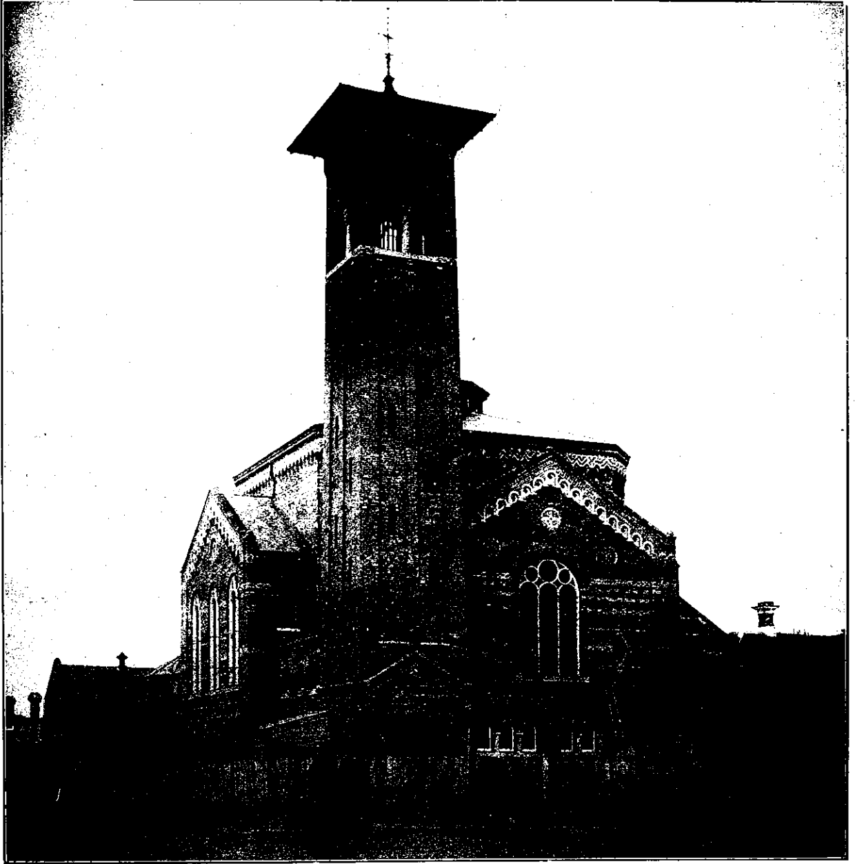
First Presbyterian Church, Invercargill, nearing completion John T. Mair, A.R.I.B.A., S.C.A. Penn., Architect, Wellington
