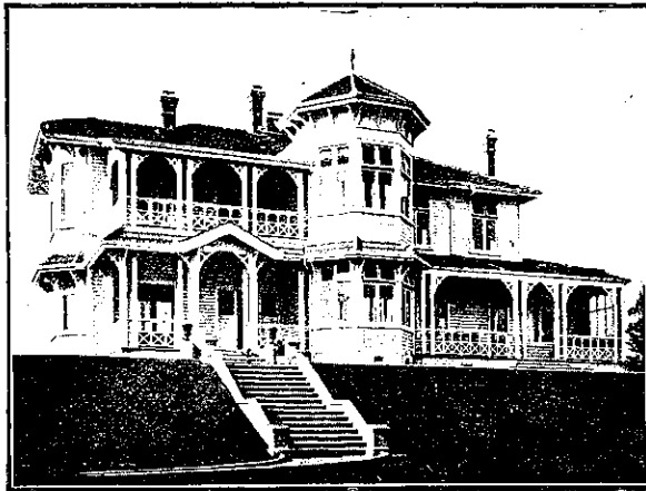
Residence for Mr. G. H. Keesing, Wanganui East T. H. Battle, Architect
