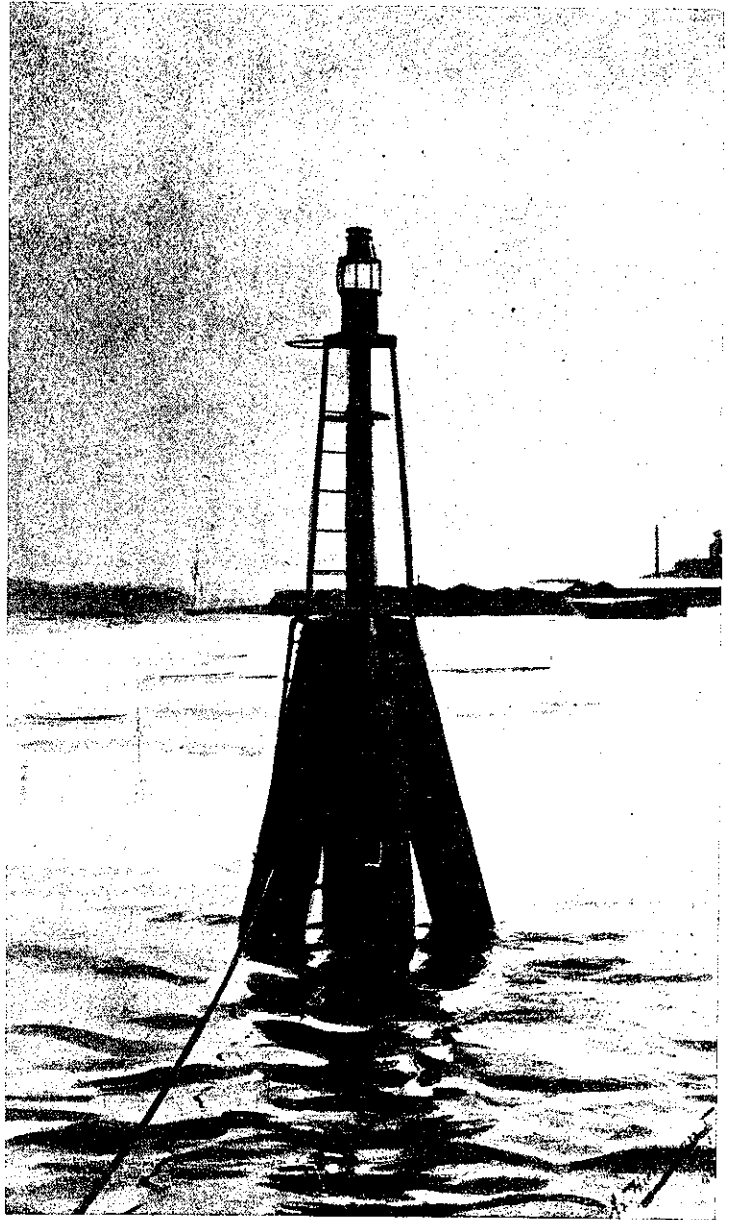
Acetone Gas Light Beacon Fitted with Flashing Apparatus
