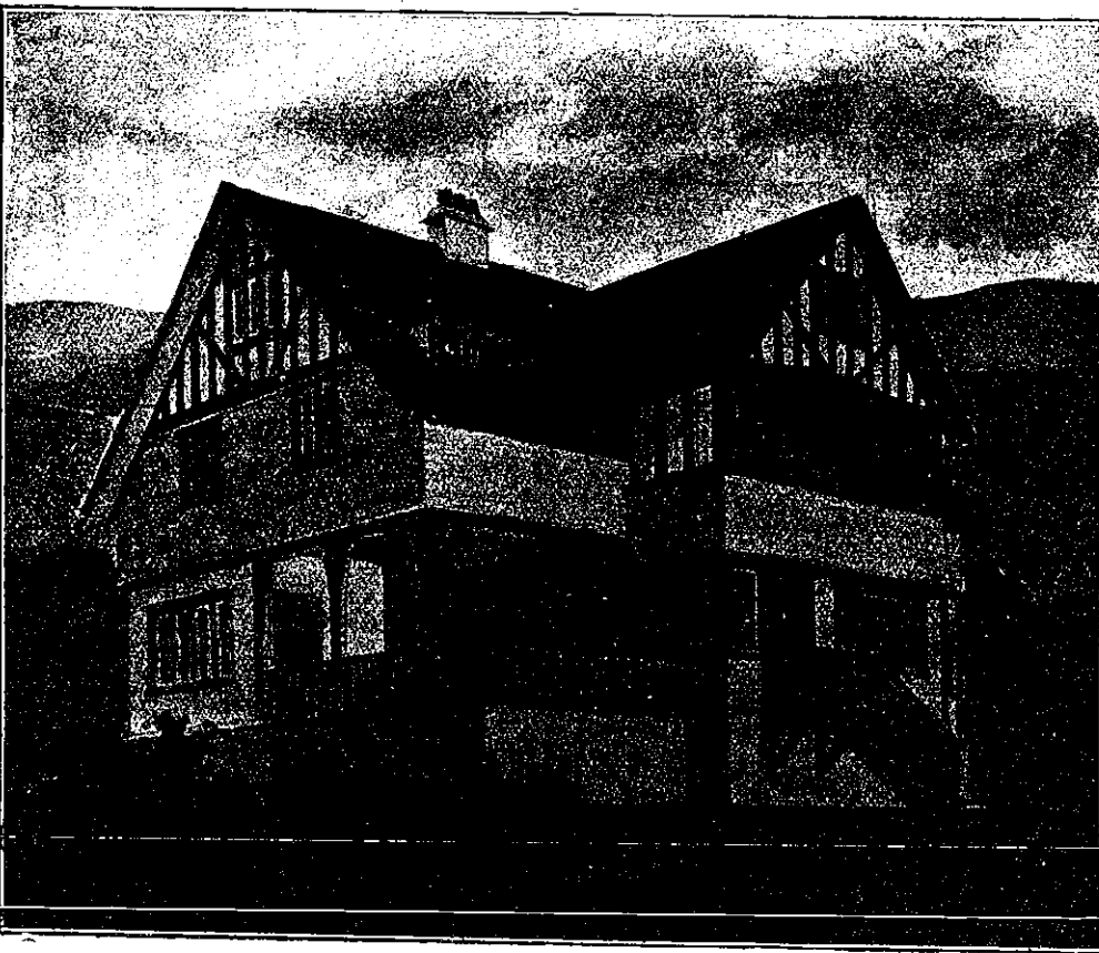
RESIDENCE IN HUTT VALLEY. F. de J. Clerc, F.R.I.B.A., Wellington.
