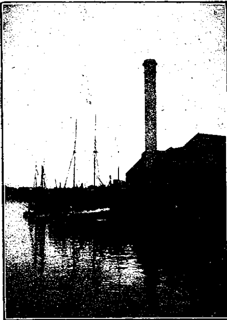
CHIMNEY, POWER HOUSE, FROM THE WHARVES.
