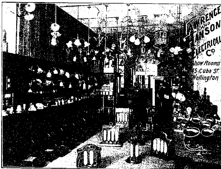
THE LAWRENCE AND HANSON ELECTRICAL CO., WELLINGTON.
