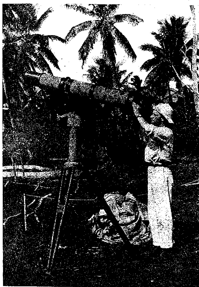
NO. 4.—THE SIX-INCH STEWARD EQUATORIAL TELESCOPE.
