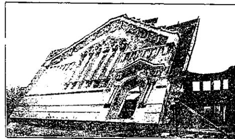
LIFTING A WALL IN PLACE BY MEANS OF JACKS.
