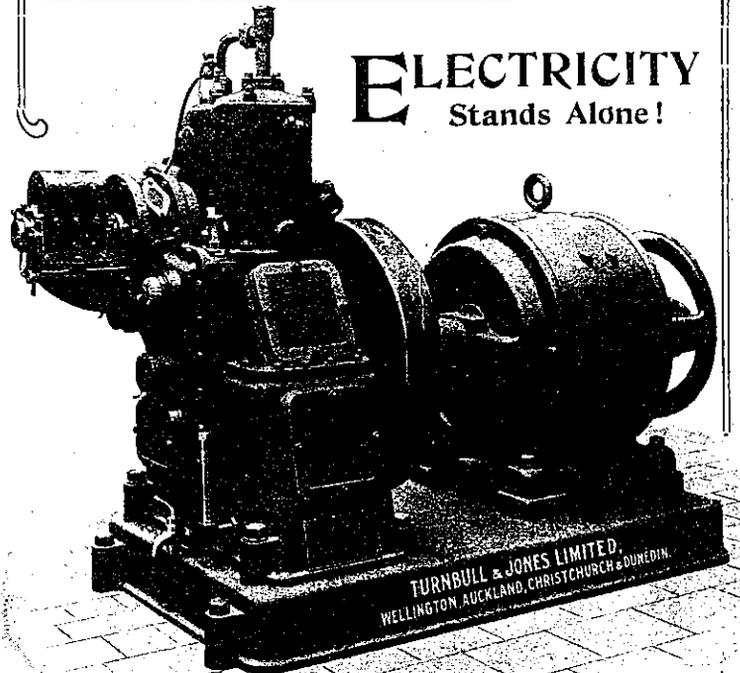
BELLIS & MORCOM OIL ENGINE direct coupled to BRITISH WESTINGHOUSE DYNAMO
