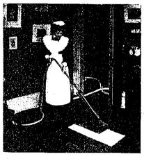
D is Hydrovakum Silent Dustman fitted outside the house. W is water pipe supplying the power. V is the valve by which the water is turned on and off. S is suction pipe with couplings C, to which the flexible hose F is attached when operating. T is the trap through which the dust is discharged into the sewer. The nozzle is passed over the carpet and the dust is sucked direct into the drain.
