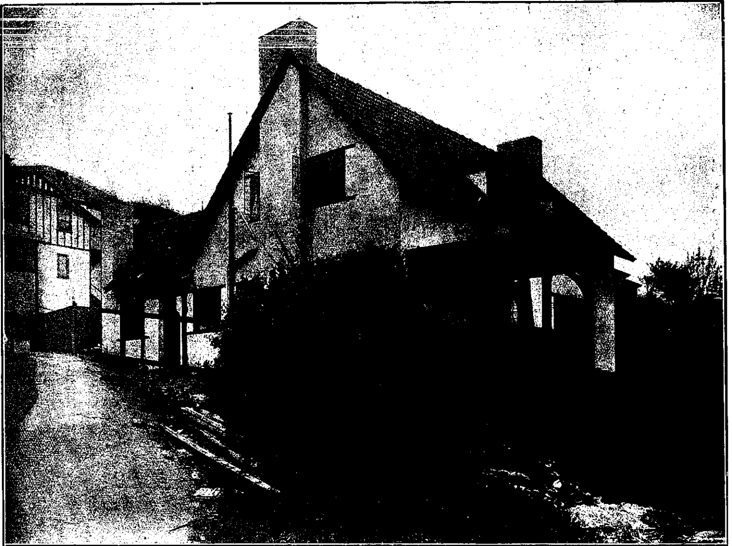
A SIMPLE COTTAGE. General View. (J. W. Chapman-Taylor, Architect.)
