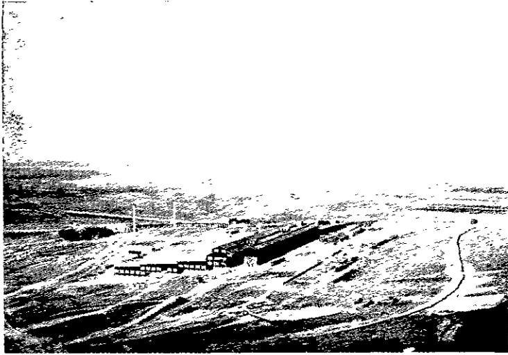
GENERAL VIEW OF GARFIELD PLANT AND WORKS
