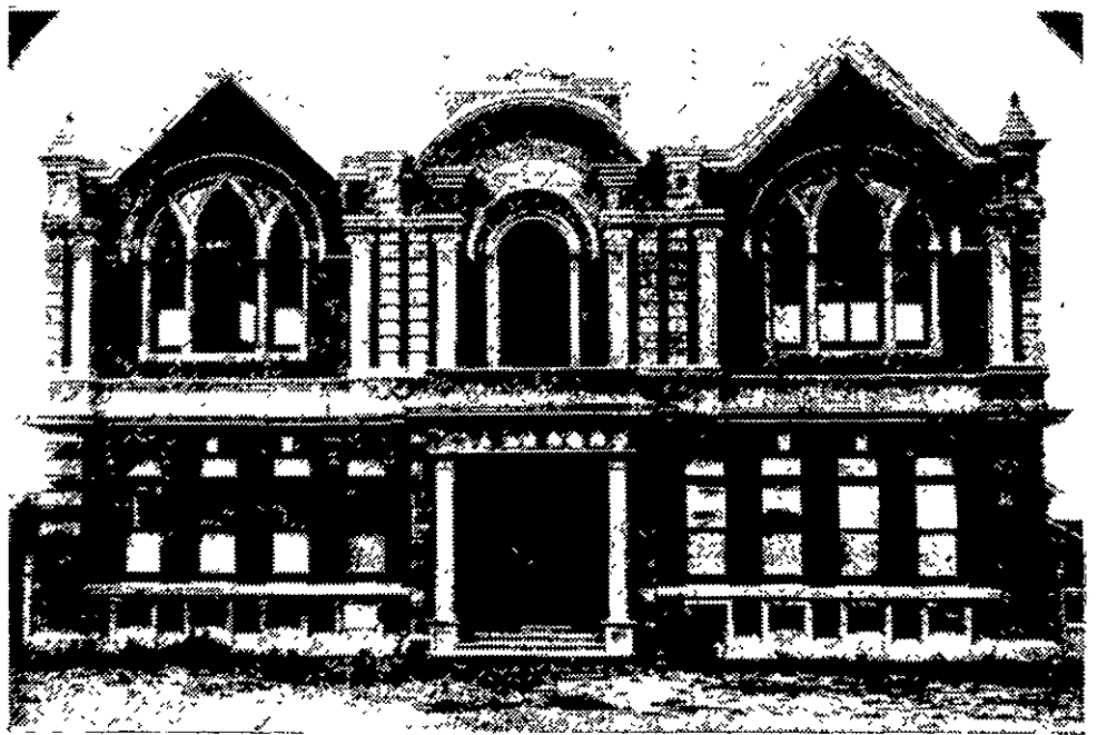
TECHNICAL SCHOOL, MASTERTON. Varnham and Rose, Architects.
