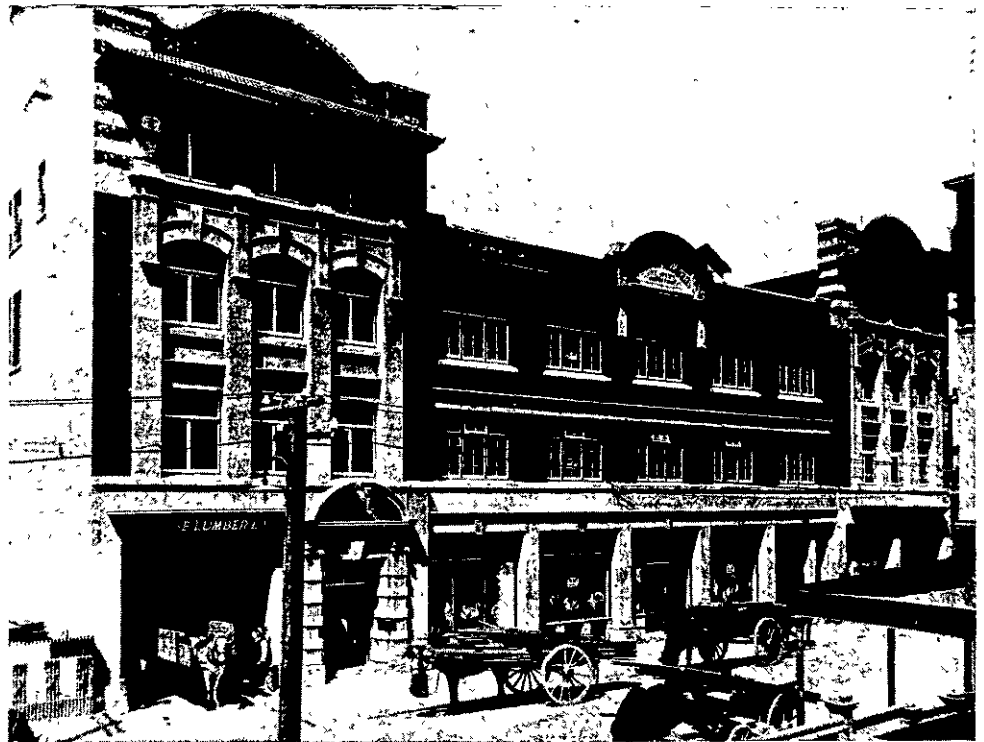
PROUSE LUMBER CO.'S BUILDING.
