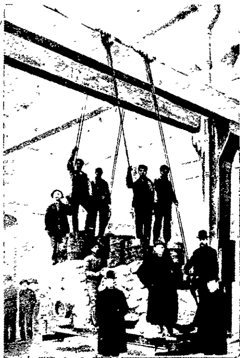
UNIQUE TEST OF REINFORCED CONCRETE.
