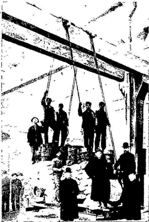
UNIQUE TEST OF REINFORCED CONCRETE.
