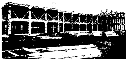
BIRMINGHAM TELEGRAPH STORES. Built of Kahn Bars throughout (Under construction.)
