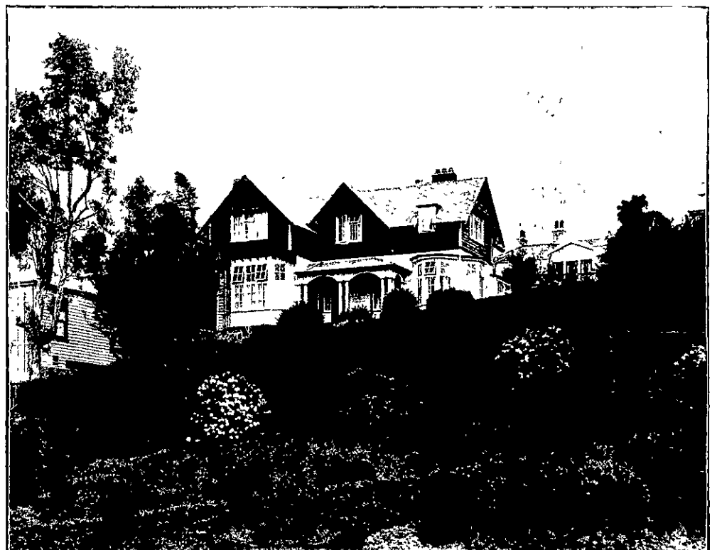
RESIDENCE, CARGILL STREET, DUNEDIN [Basil Hooper, A.R.I.B.A., Architect.]
