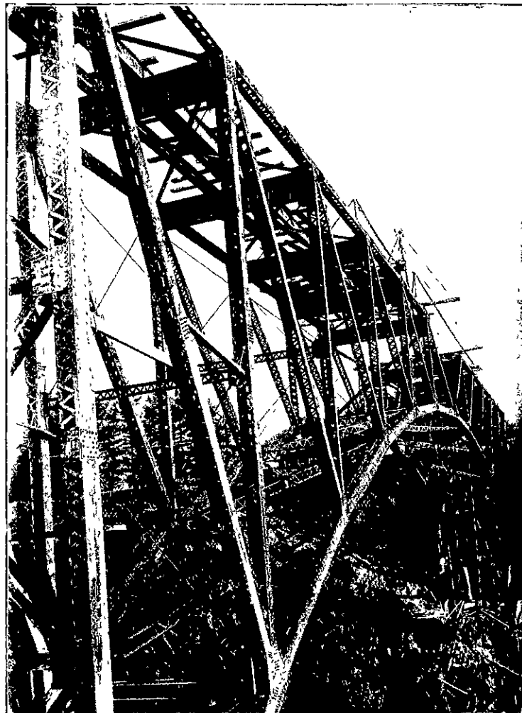
CAMBRIDGE BRIDGE: THE COMPLETED ARCH.
