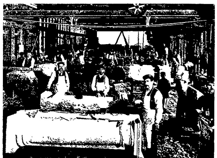
STONECUTTERS' SHED (STOUT STREET).
