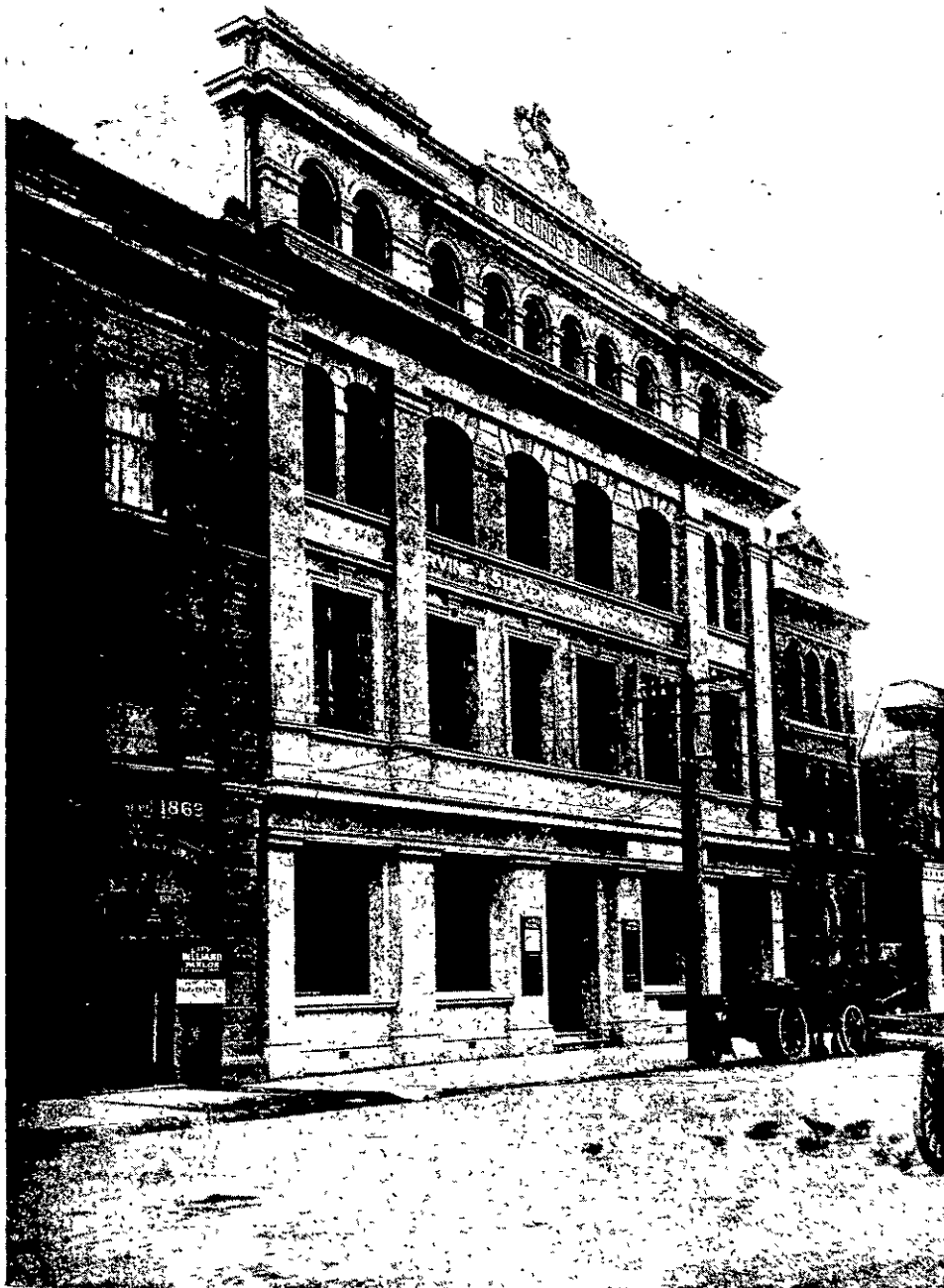
ST. GEORGE'S BUILDINGS, BRANDON STREET, WELLINGTON. [Architects, Crichton and Mackay]
