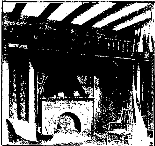
MR. EWEN'S CHIMNEY CORNER (Contractors, Brown and Johnston.)
