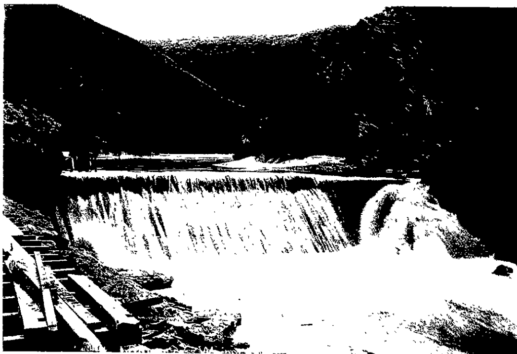
THE DAM ACROSS THE WAIPORI RIVER.
