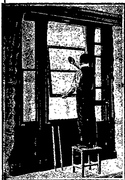
TOP SASH, SWINGING FOR CLEANING.
