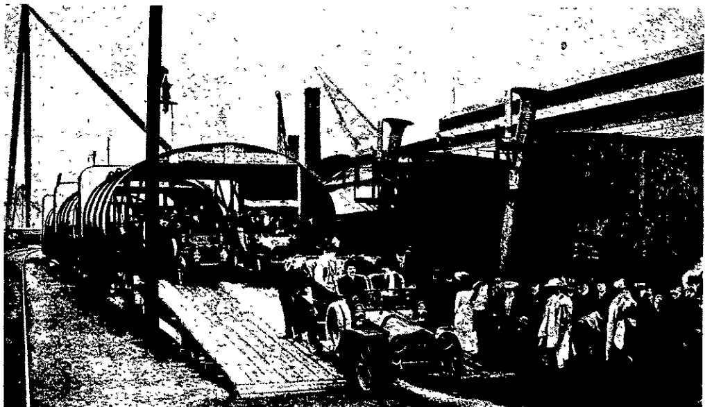
AT WALLSEND-ON-TYNE AT THE RECENT LAUNCHING OF THE FIRST OF THE GREAT CUNARDERS, THE "MAURETANIA," A NOVEL DEMONSTRATION WAS GIVEN. THREE OF HER FOUR OVAL FUNNELS, WHICH ARE 17 FT. 6 IN. X 23 FT. IN., AND WHICH TOWER 120 FT. ABOVE HER LOAD WATER LINE, WERE LAID IN A ROW, AND FORMED A HUGE TUNNEL THROUGH WHICH MOTOR CARS WERE DRIVEN TWO AHEAD.
