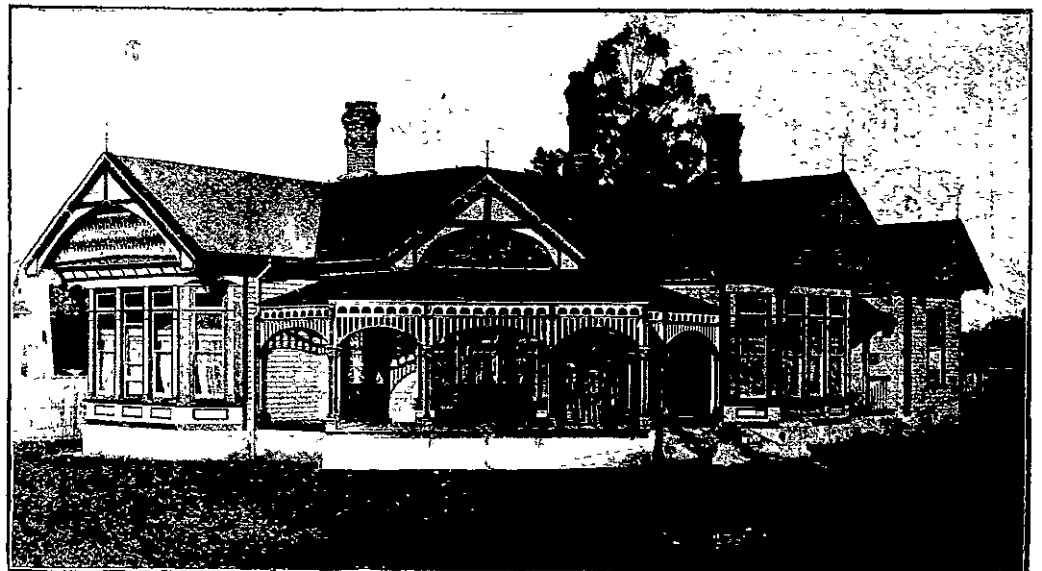
TYPICAL CANTERBURY HOME (DR. BRITTIN'S HOUSE, CHRISTCHURCH)
