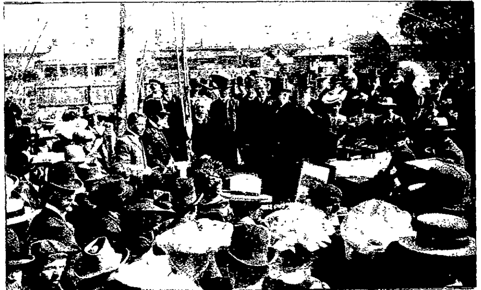
SIR JOHN GORST LAYING THE FOUNDATION STONE.
