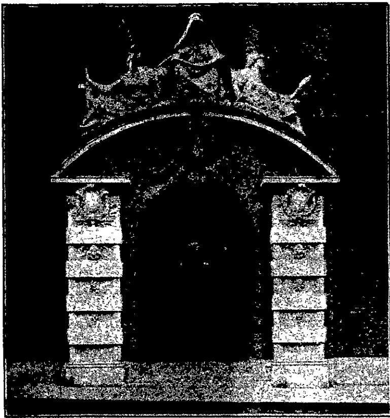
CENTRAL CRIMINAL COURT: ENTRANCE GATE.
