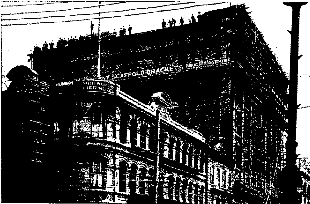
HUMPHRIES' PATENT SAFETY SCAFFOLD BRACKET IN USE ON MESSRS. JOSEPH NATHAN AND CO.'S NEW BUILDING, WELLINGTON.
