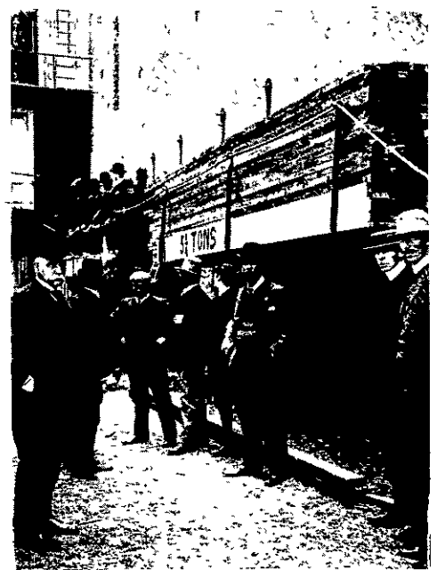
TEST OF THREE BRACKETS ON SIDE WALL OF THE PIER HOTEL, WELLINGTON, LOADED WITH 5½ TONS OF RIMU, WHICH WAS CARRIED EASILY.
