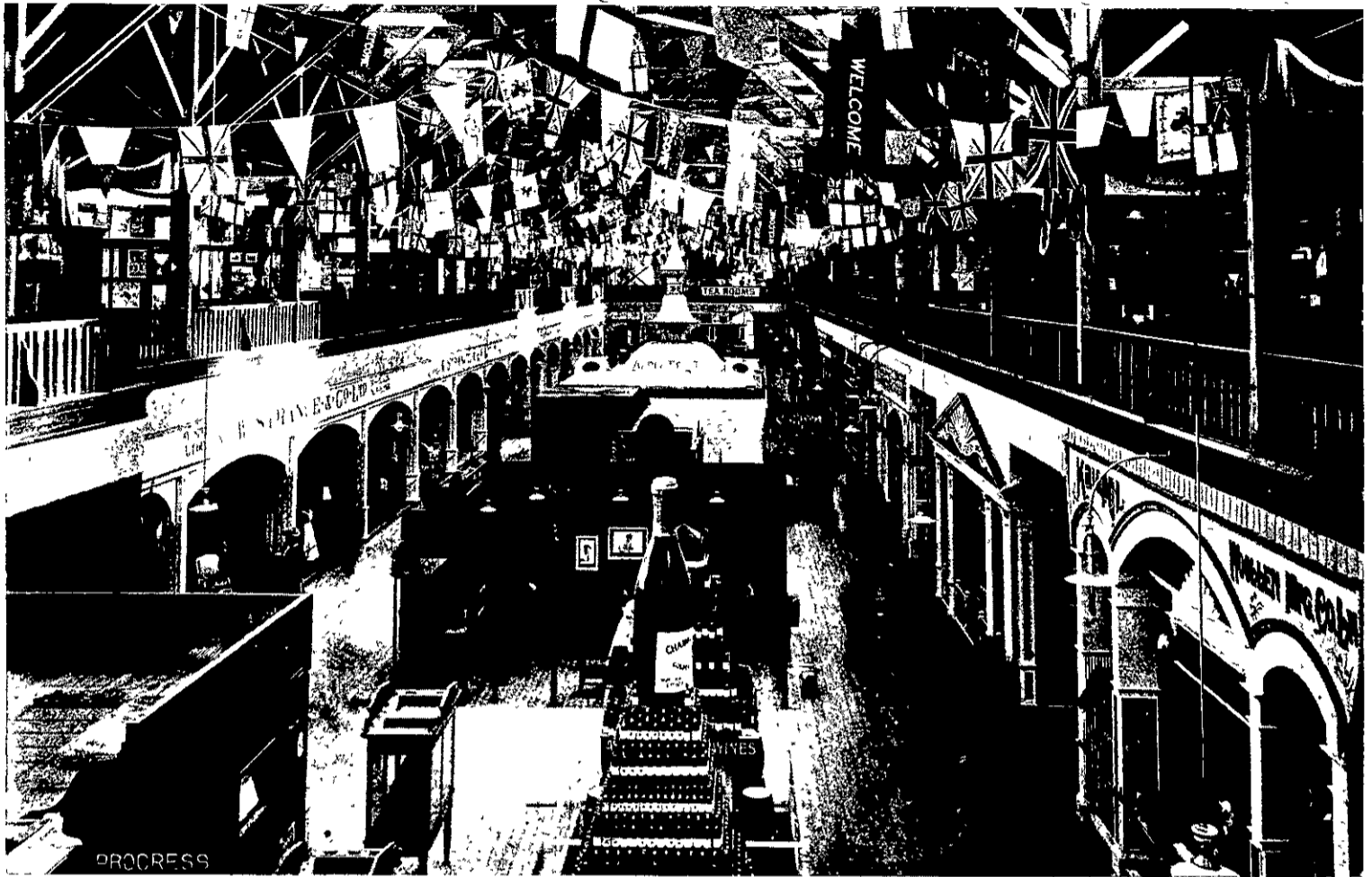
A GLIMPSE AT THE NORTH WING, MAIN BUILDING.
