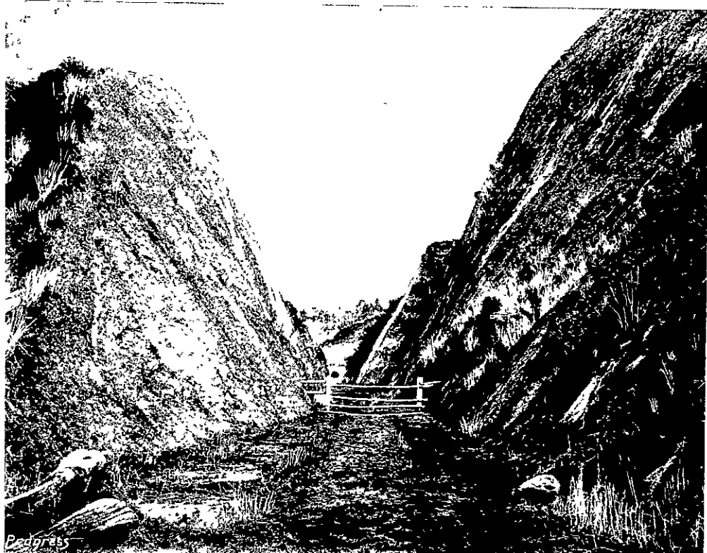
NORTH ISLAND MAIN TRUNK RAILWAY: MANGAWEKA SECTION—A PAPA CUTTING.
