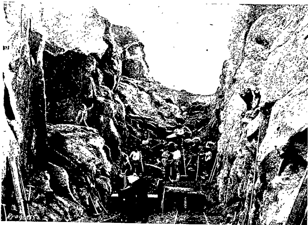
NORTH ISLAND MAIN TRUNK RAILWAY: OHINEMOA SECTION—A RHYOLITE ROCK CUTTING.
