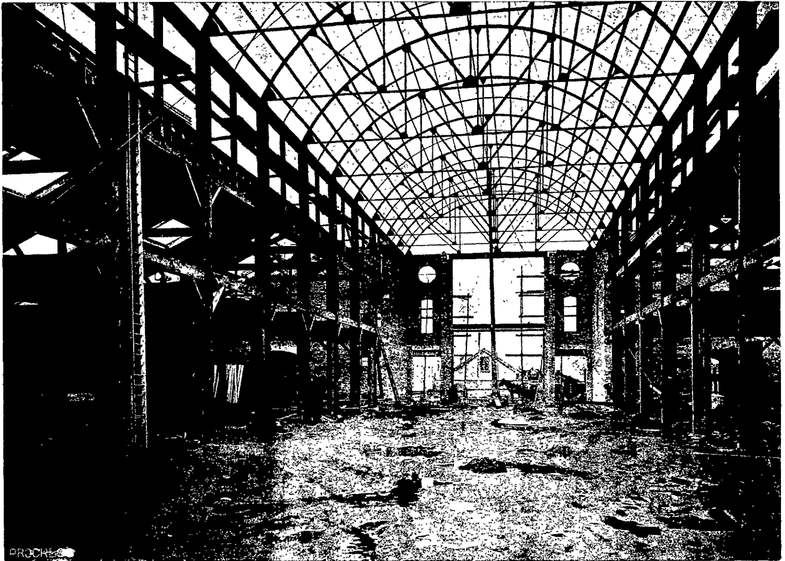
INTERIOR OF THE FARMERS' SALEYARDS BUILDING, CHRISTCHURCH.
