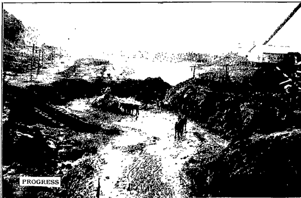
EXCAVATIONS AT THE NEW PORT CHALMERS DOCK.
