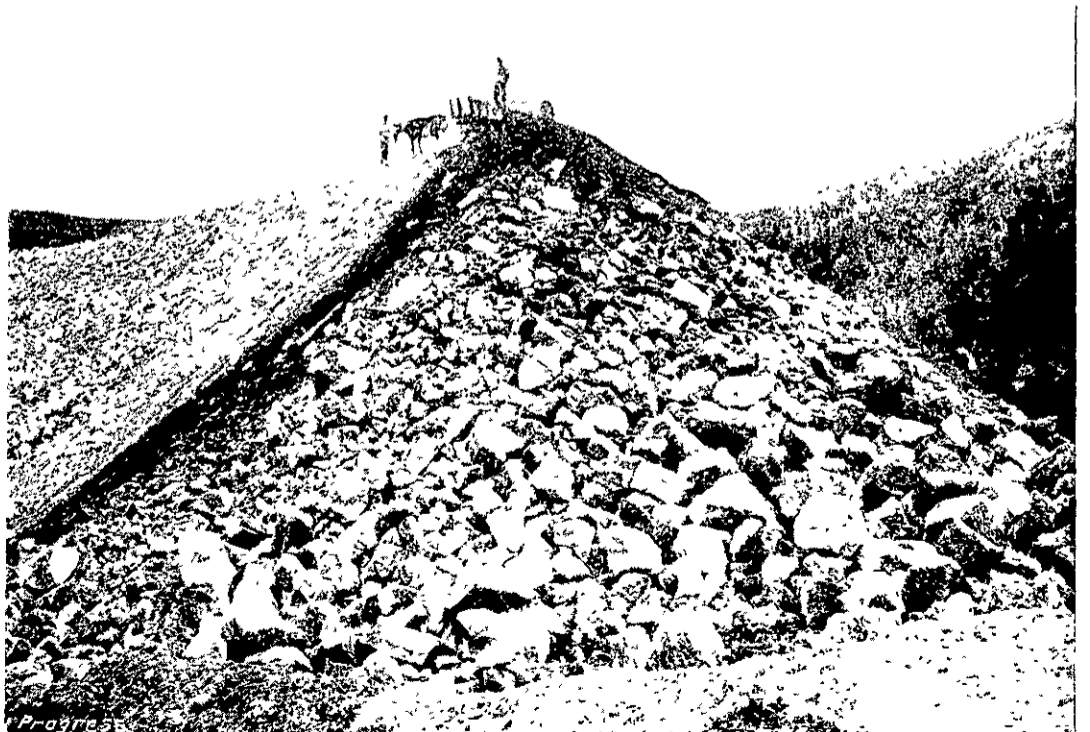
NORTH ISLAND MAIN TRUNK RAILWAY OHINEMOA SECTION—BANK FORMED OF RHYOLITE DEBRIS.
