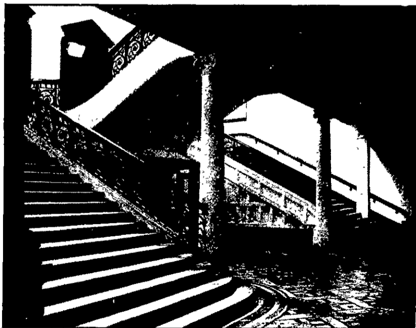
GRAND STAIRCASE, WELLINGTON TOWN HALL.
