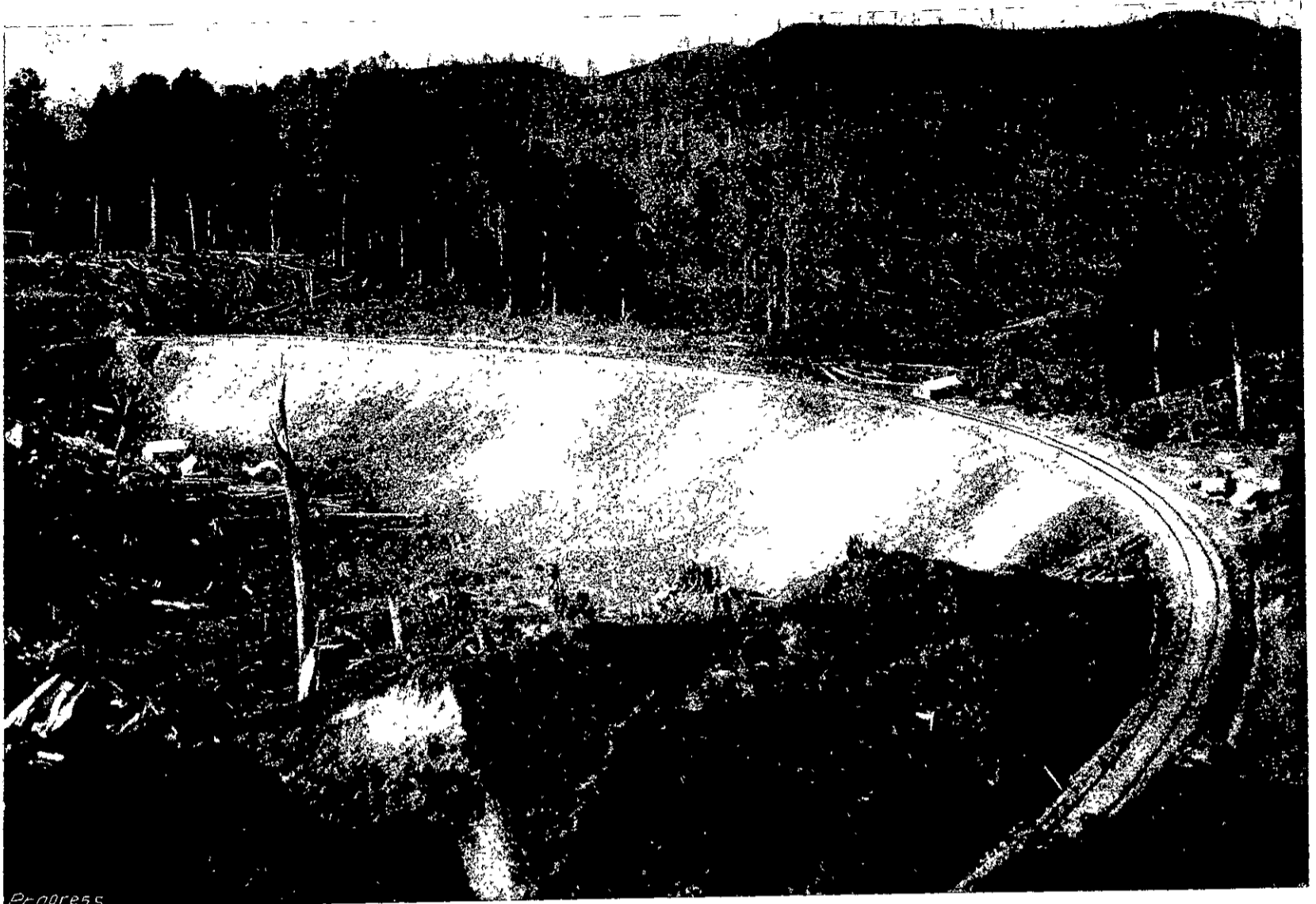
EMBANKMENT, about 2 miles north of Taihape, 63 ft. high; contents, 100,000 cubic yards.
