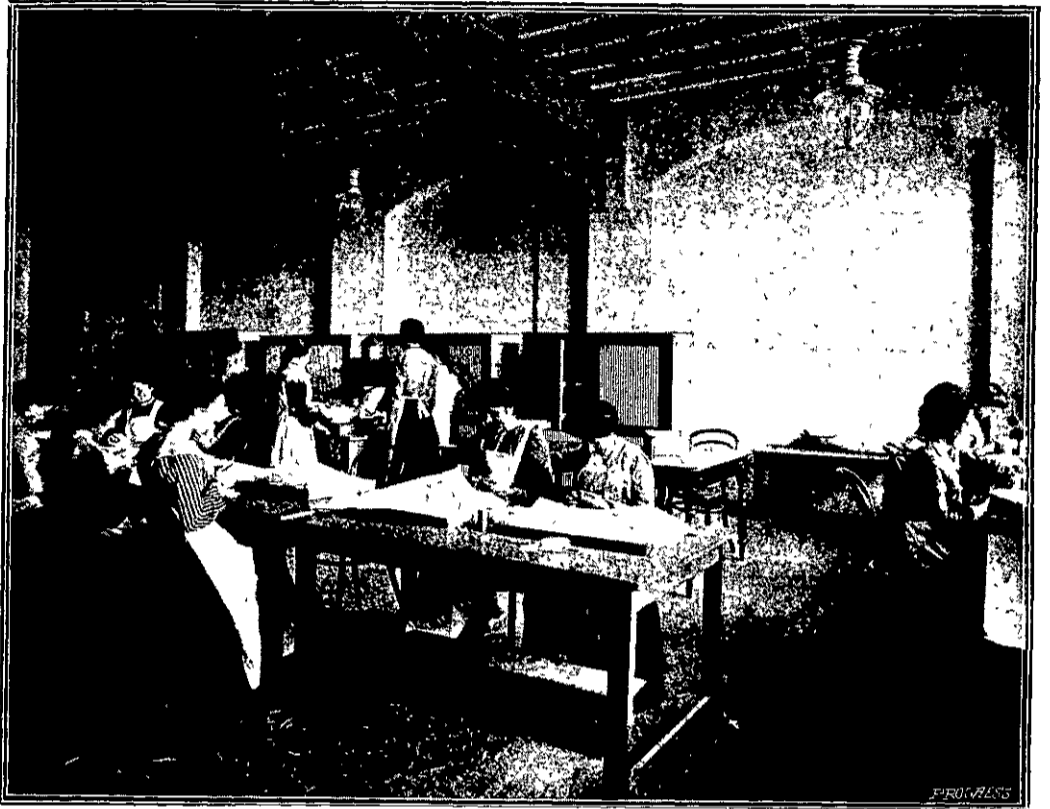
IMPREGNATING AND SEWING THE MANTLES.
